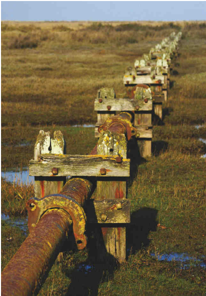
The chemistry of corrosion worldwide can affect thousands of miles of metal piping for water and petroleum products. (Picture courtesy of Owens Corning.)
