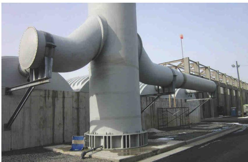
*For a New Jersey odour control system, FRP ductwork built by ECS using AOC Vipel vinyl ester resin and Owens Corning glass helps move 3400 m³ per minute of air and saved the end user 60% in component costs compared to stainless steel equipment.*
