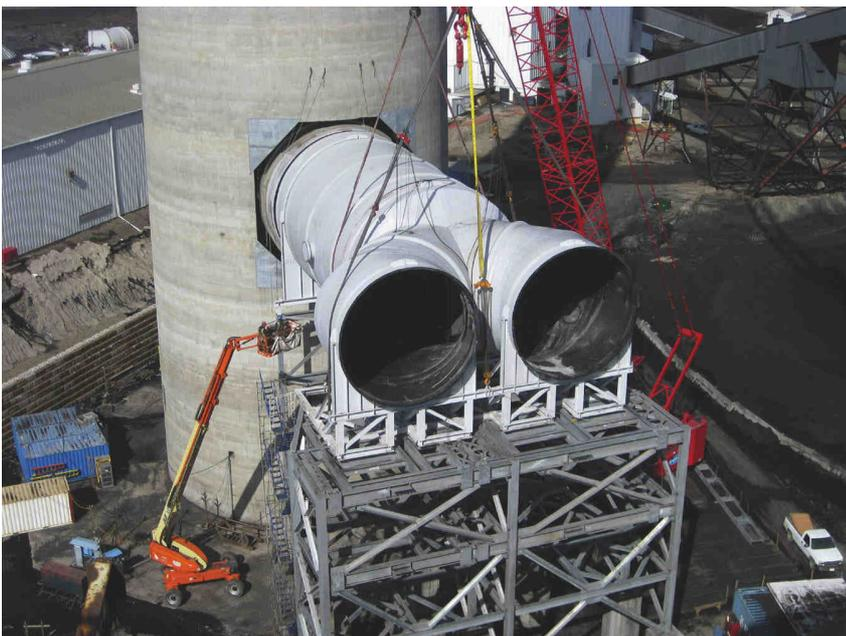
*That's no Space Shuttle exhaust, that's large spool FRP ductwork made with Ashland's HETRON epoxy vinyl ester resin and glass for a North Dakota FGD system. Ershigs filament wound the 21-30 ft diameter components.*
