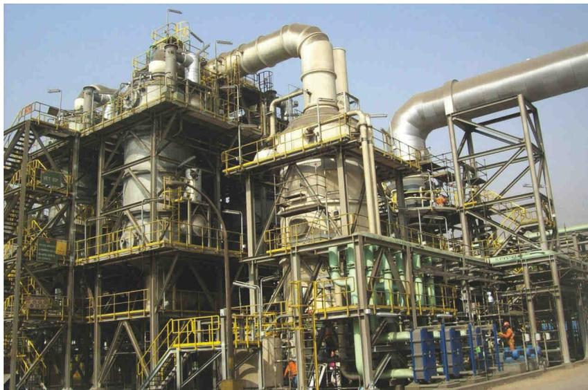
**Minerals processing is a growth area for FRP. At the sulphuric acid plant that is part of Votorantim Metals' zinc refinery in Cajamarquilla, Peru, FRP scrubbers, tanks, piping and ductwork are made using Ashland's Derakane epoxy vinyl ester resins.**
