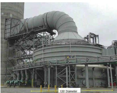
*Success story for FRP: Ashland's glass-reinforced resins offer corrosion protection in the scrubber and ductwork equipment that is part of one of the largest jet bubbling reactors in North America, installed at a 950 MW power plant.*
